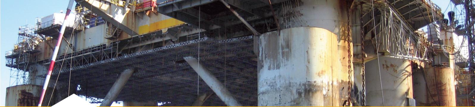
By placing compressors, generators, welding and cutting plant on the QuikDeck temporary decks, your teams have greater space for execution – reducing the constant shifting of equipment and aiding in the productivity.
